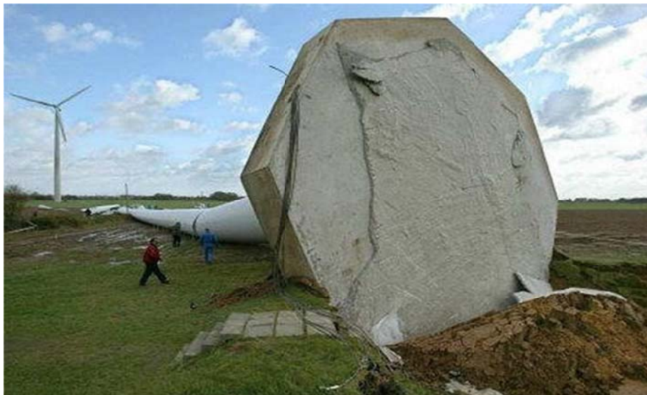
Figure 5: Fallen Turbine
