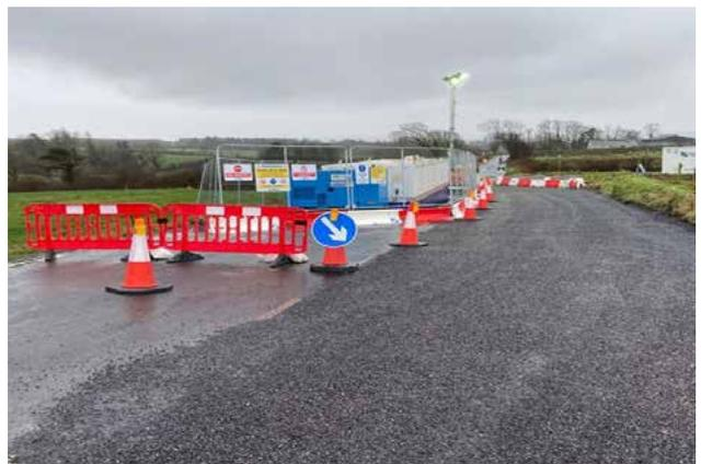
**Figure 8: A typical passing bay in operation during cable jointing**
