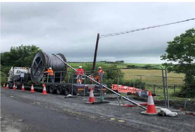
**Figure 7: Cables being pulled into the ducts and jointing bay**
