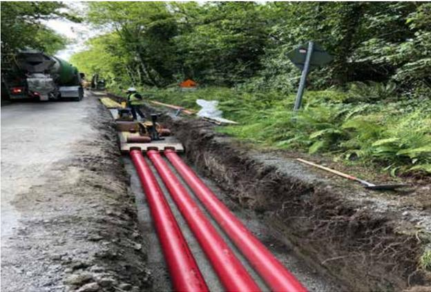
**Figure 5: A typical cable duct installation in the road**
