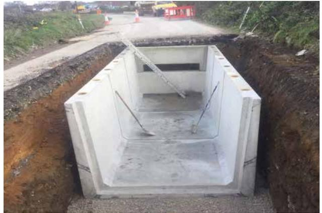
**Figure 6: A typical jointing bay where cables are connected**
